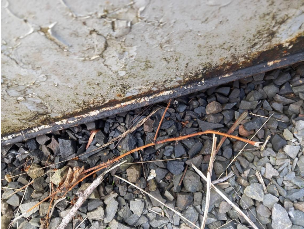
Photograph 9: Diesel tank leak at northeast corner
