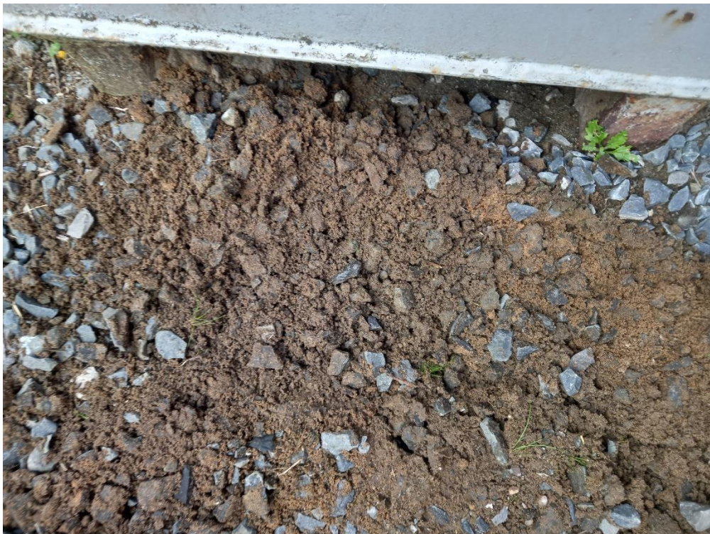
Photograph 10: Sand subsurface to the gravel ground cover within the storage area
