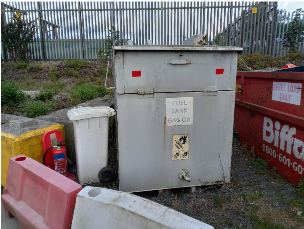
Photograph 8: Large (3,500 litre) steel diesel tank within storage area
