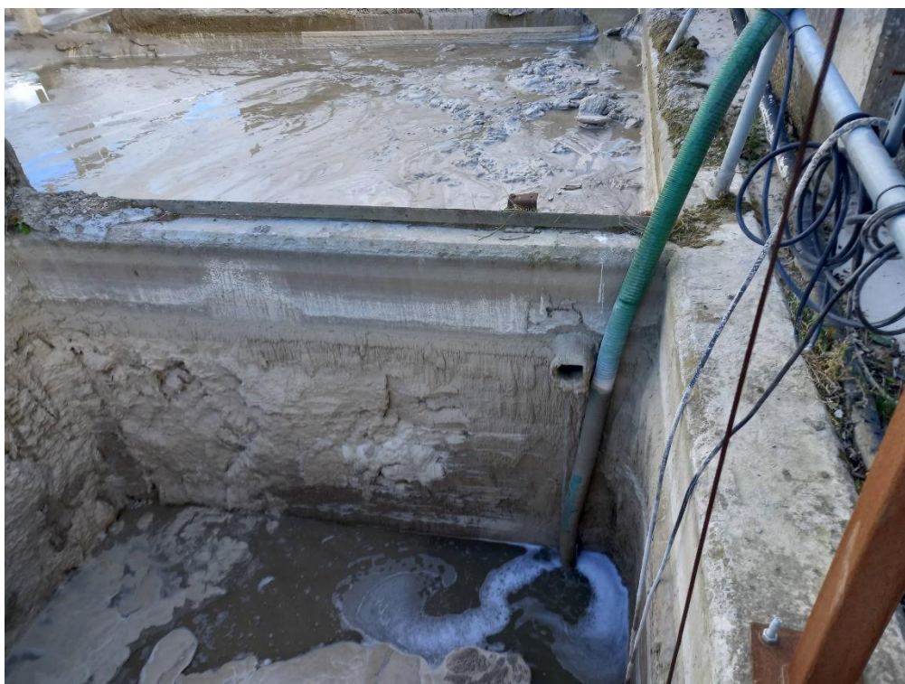
Photograph 22: An overflow pipe allows for excess water to discharge into a deeper dug out trench
