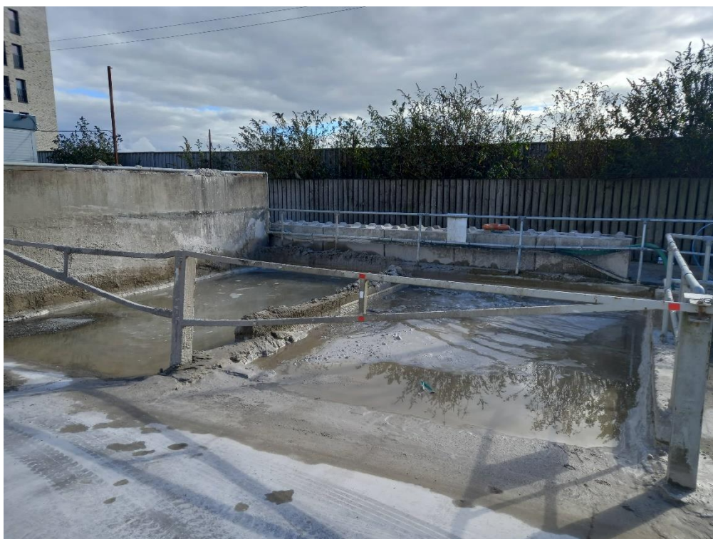
Photograph 20: Onsite concrete washout area
