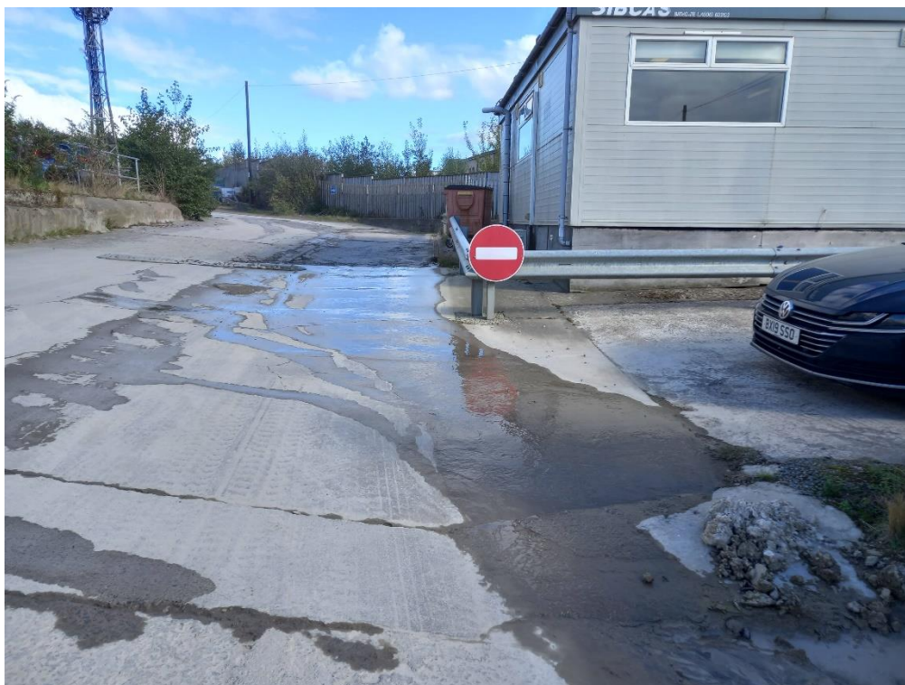
Photograph 21: Surface water runoff from the batching facility
