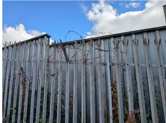
Photograph 16: Steel palisade fence.
